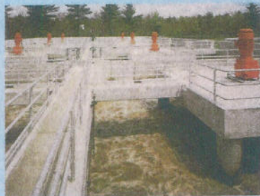
Mechanical aeration tanks
