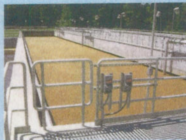
Diffused air aeration tanks
